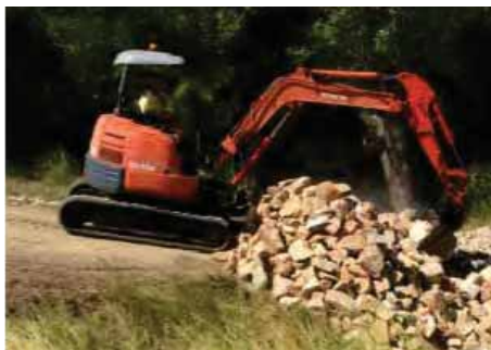
Earthworks at Gympie Sporting Clays
